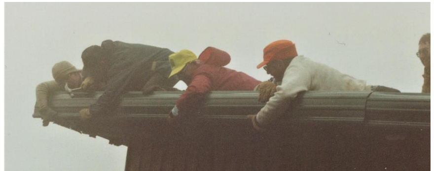
Replacing the roof on Cooper Lodge inside a cloud in the early 1980s.
