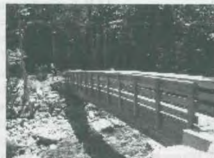
The new Old Job Bridge. Massive wooden girders!
