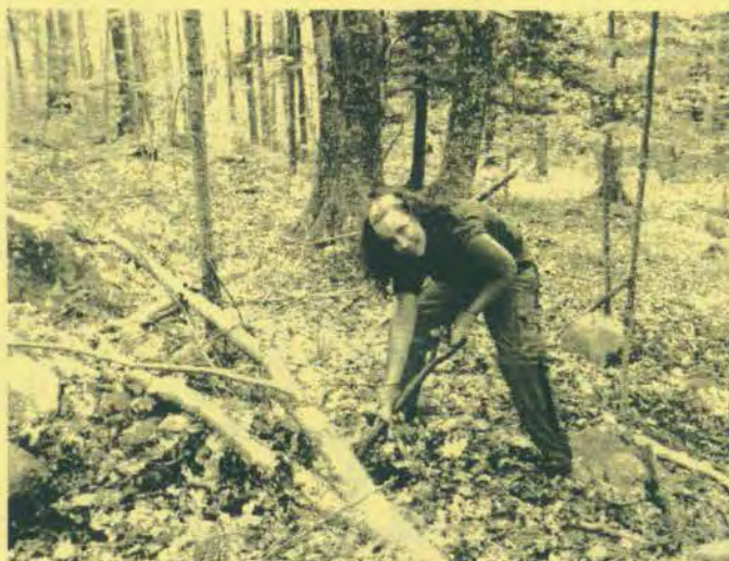
Hoeing Out a Water Bar
