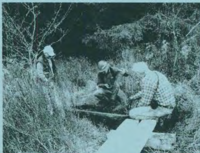
Killington Section members installing puncheon
